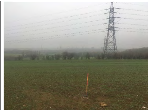
Plate 3 – Looking W downslope towards the steelworks from the substation area.
